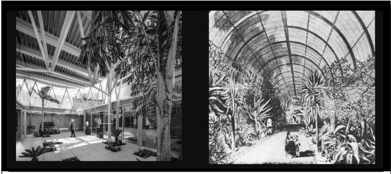
Figure 3: Extracted from the visual presentation at ACSA conference. On the right, Chatsworth Greenhouse by Joseph Paxton in 1836. On the left, The Tobogan House by Z4A, Madrid, Spain, 2016.
